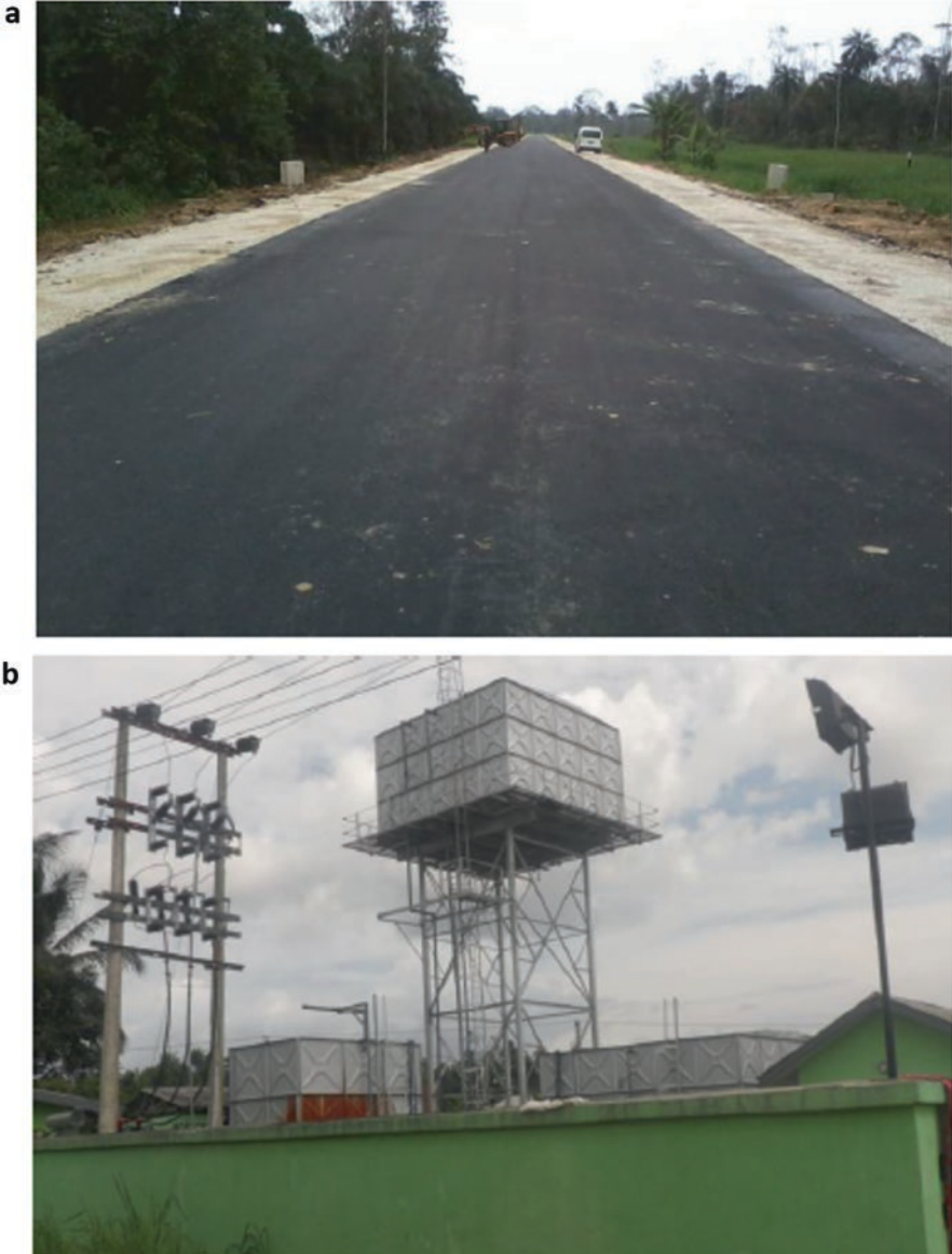
Fig. 14.6 (a) 4 km road built between Shell's facilities and Gbaran host communities (Gbaran/Ekpetiama cluster). (b) Water tower for the Gbarantoru community (Gbaran/Ekpetiama cluster). (c) Power station for Obunagha and Gbarantoru communities (Gbaran/Ekpetiama cluster). (d) 18-classroom block in Onopa community (Epie/Atissa cluster) (Source: Shell)
